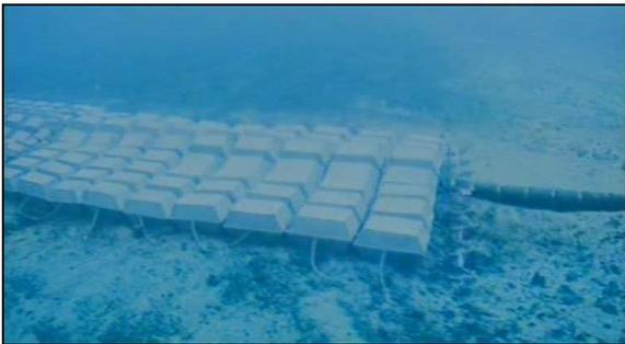
Figure 5 – Concrete Mattress over a Pipeline
