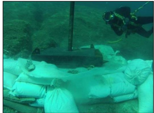
Figure 6 – Diver Installed Grout Bags
