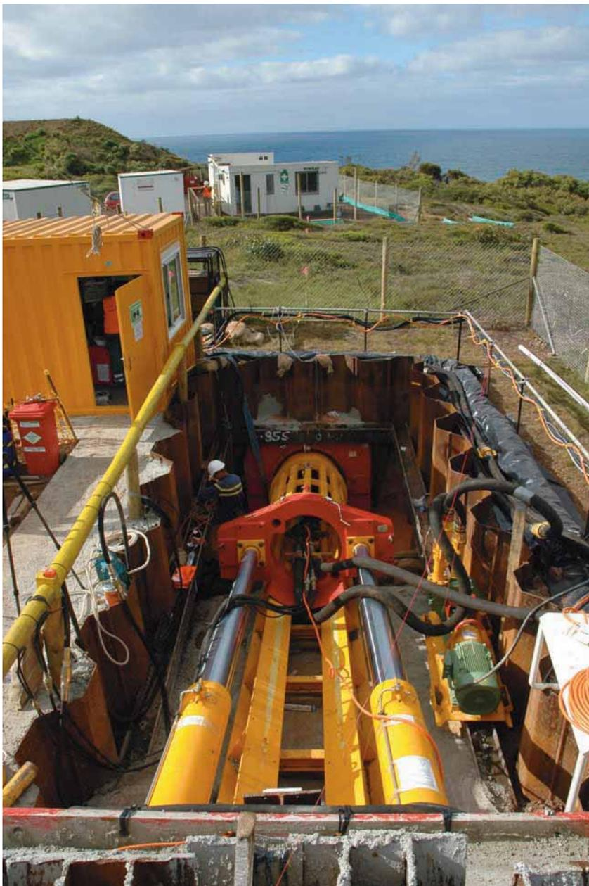
Figure 4. Microtunnelling site at a pipeline shore crossing.
