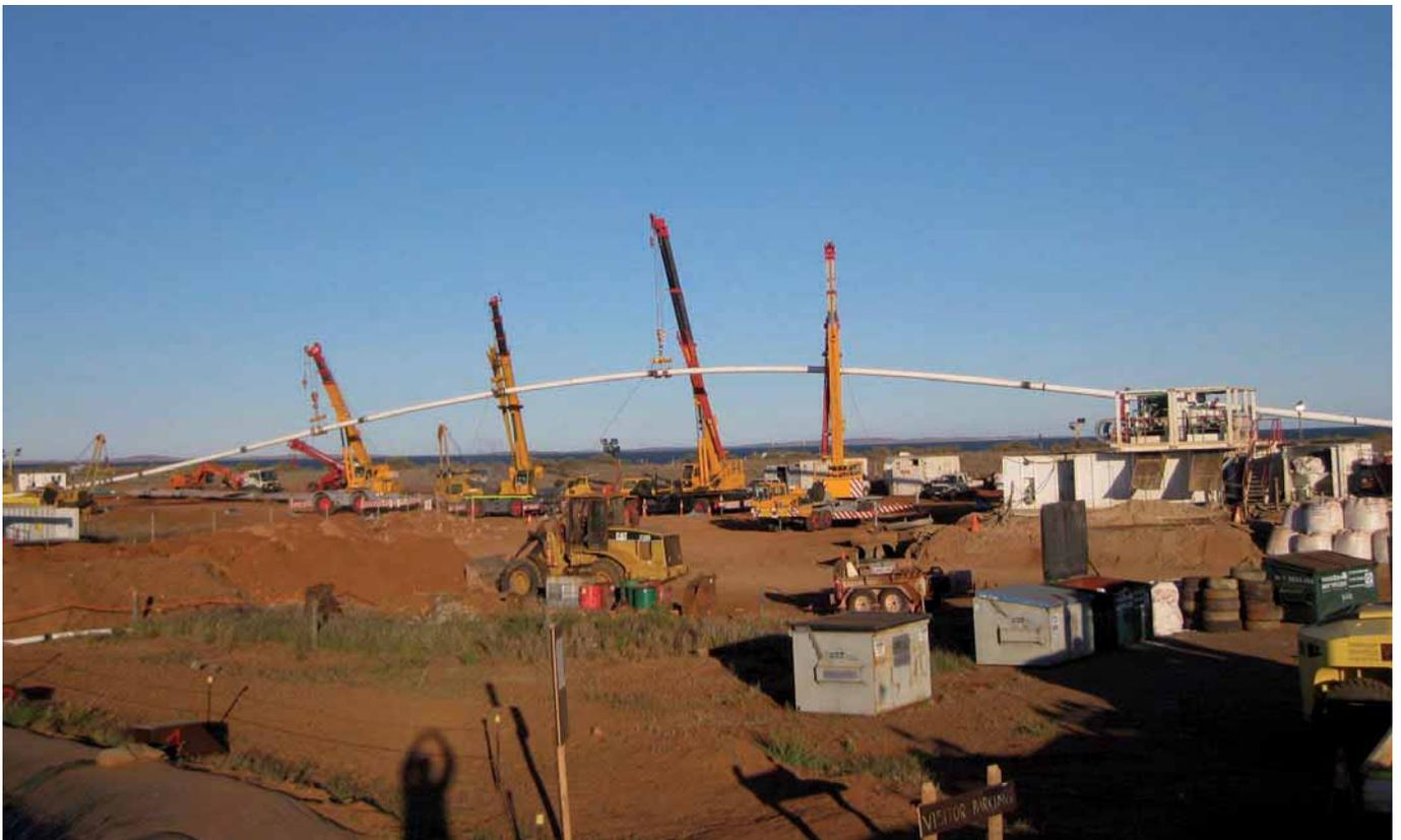
Figure 3. Pipeline installation at shore crossing by HDD.
