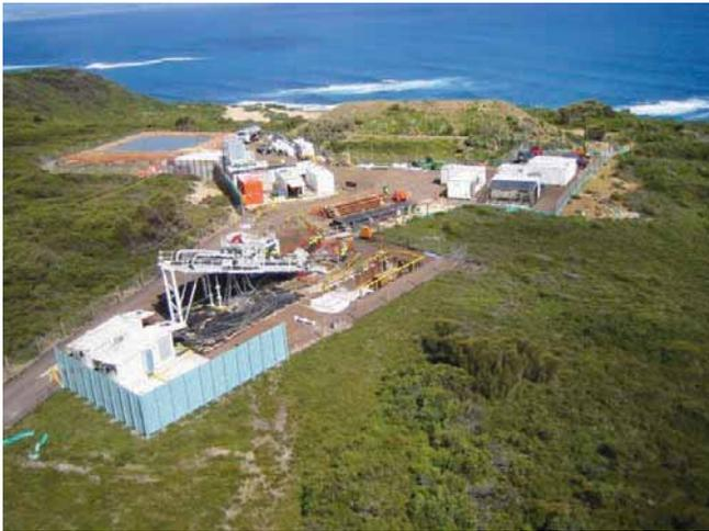
Figure 2. HDD set-up for a pipeline shore crossing.
