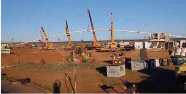
**Figure 2.** The pipeline over-bend for the forward thrust installation.
