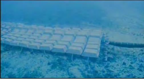
Figure 4 – Mattress over a pipeline
