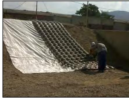
Figure 2 - Mattress placement on slopes
